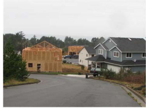
N.E. 71st and Avery Housing Construction
