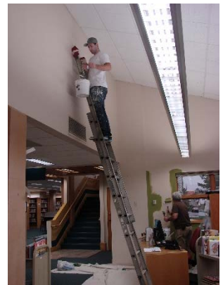
Newport Library Renovation
