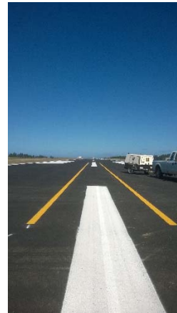
Airport Runway Reconstruction
